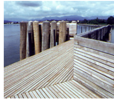
Abb. 6.01: Steganlage in Rapperswil-Hurden (CH)
